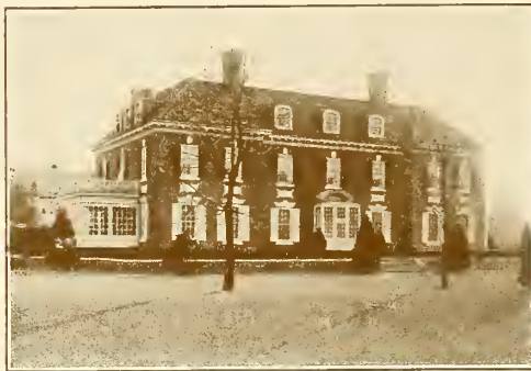
Residence of CHAS. A. PORTER, JR., Philadelphia Horace Trumbauer, Architect
